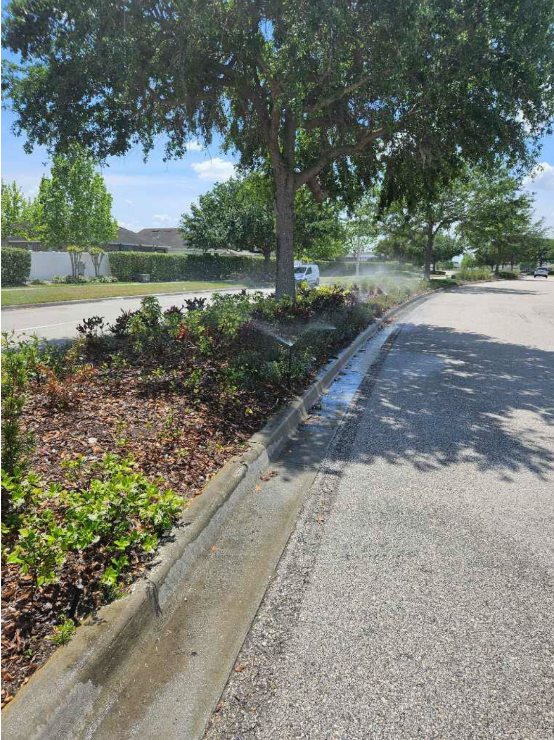
New 12" pop-ups installed in center island of Ayersworth Glen.
